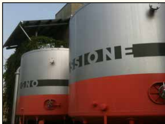
Figure 37. Cisterns at Pearl Brewery in San Antonio capture roof runoff for landscape irrigation.
