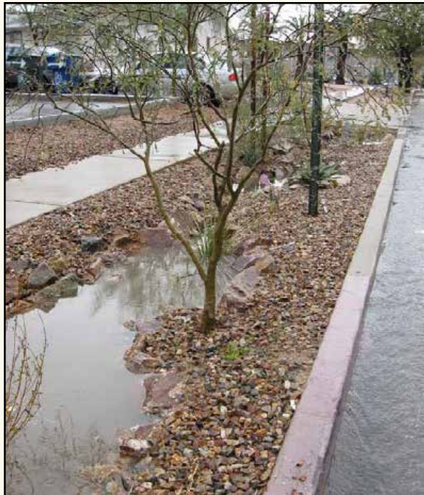
Figure 30. Roadway biofiltration planter located in street right-of-way, Tucson AZ.
