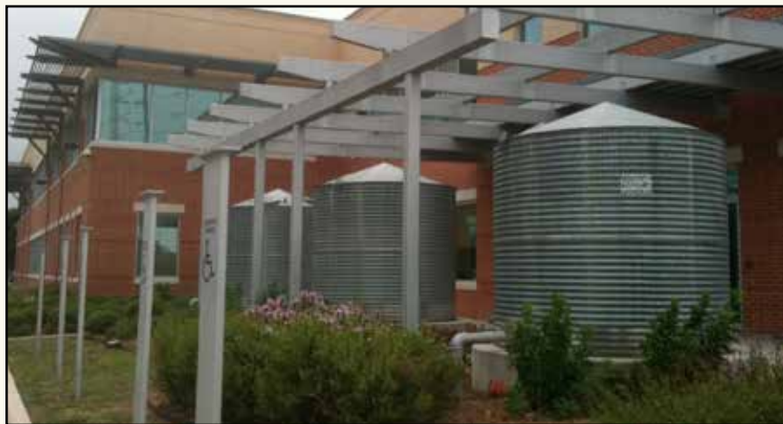
Figure 36. Cisterns capture air conditioning condensate for reuse, San Antonio city administration building.
