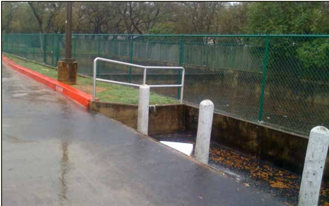
Figure 14. Sand filter, the most common BMP in the Austin-San Antonio region (Photo by Annalisa Peace, GEAA website, 2010).
